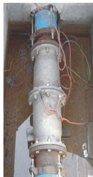
150mm Care-Free Conditioner turns over entire lake every 36 hours. Flowrate 6,000 lit/min.
